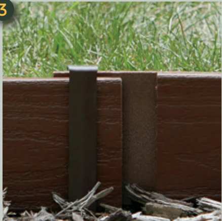
Hammer the stake until it is flush and over lapping both boards.
