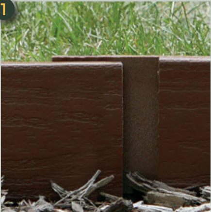
After clearing a level path, lineup the edges with a 1.25 inch gap.
