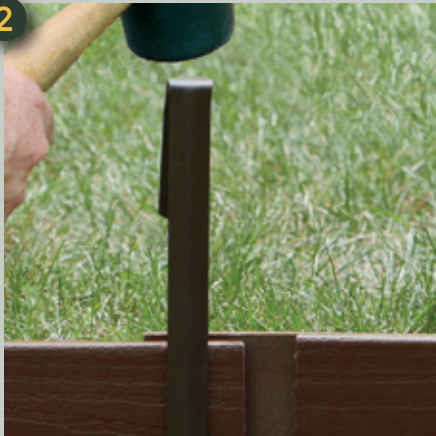
Hammer in the stakes. Make sure the hook is overlapping the two.
