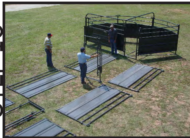
Stand up the ADJUSTABLE ALLEY FRAME (G) to begin alley installation.
