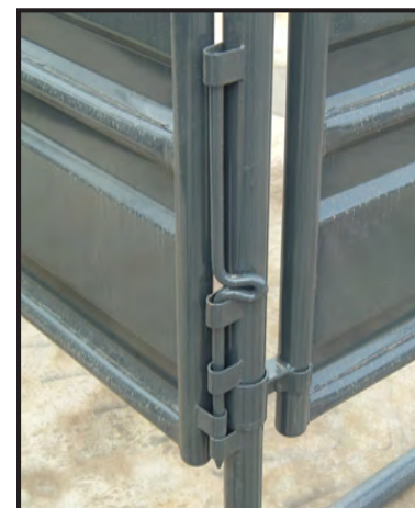
Connector pin. This is only at the pivot point of sweep.
